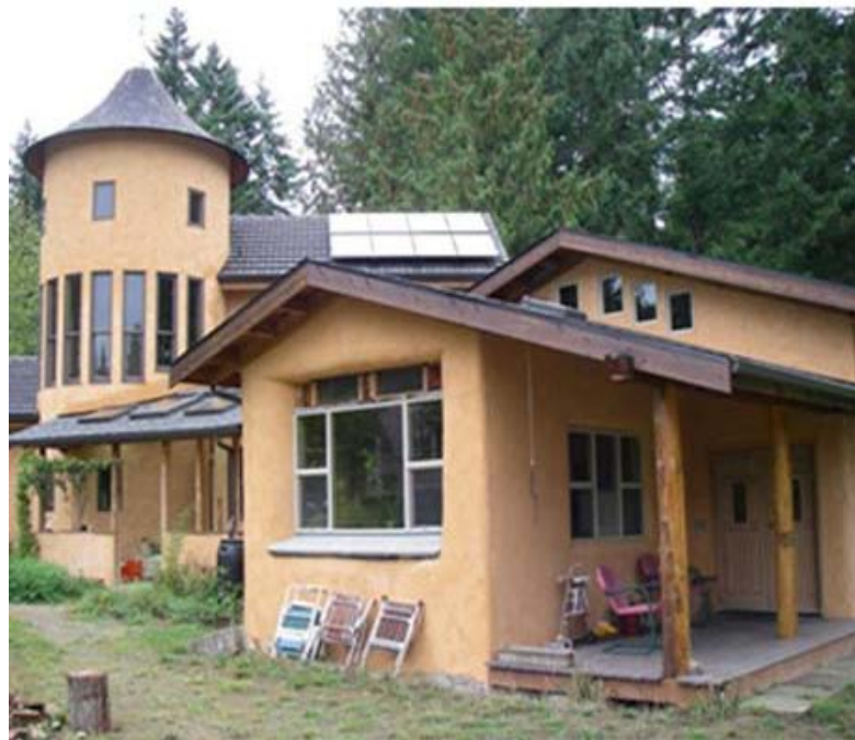
Photo: Top, a straw bale home being constructed; bottom, a completed straw bale home
