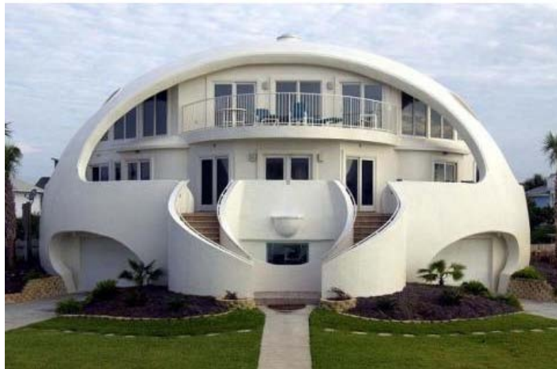
Photo: Top left, a modern geodesic home; top right, the frame of a dome house before the panels have all been added; bottom, a dome constructed of concrete. This particular dome is of interest because it survived a direct hit by hurricane Ivan in 2004 and survived virtually unscathed
